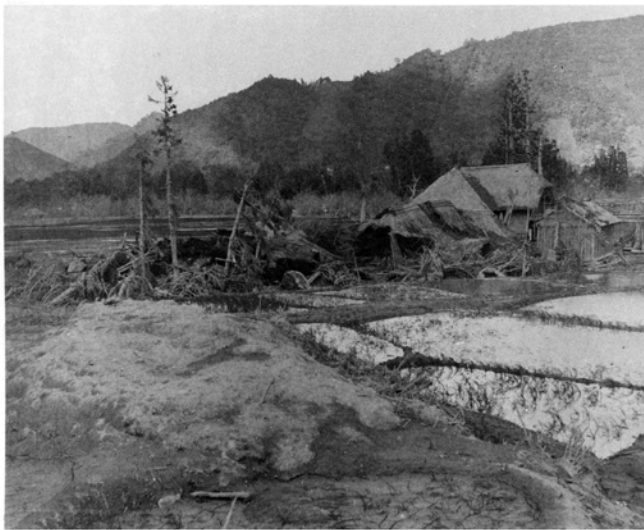
第 15 図 宮内庁所蔵、整理番号 56. 「颶風渋谷村民家ヲ破壊セル図」 Fig. 15 A photograph from the possession of the Imperial Household Agency. Reference number 56. "The photograph of a private house in Shibutani-mura destroyed by strong wind".
